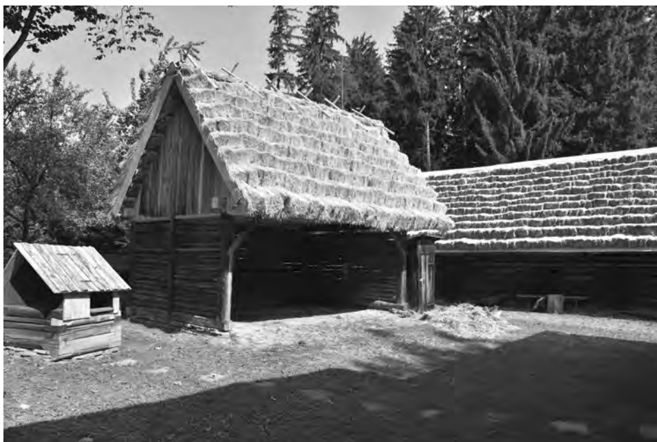
Fig. 1, 2. Open shed and combined outhouse of the farmstead from Vyšný Kubín before and after reconstruction. Photograph by R. Sýkora, 2018
